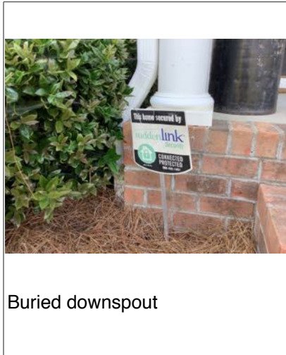
Gutters appear to empty into flowerbeds near homes foundation.
